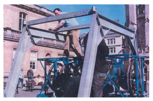
23. Pass-up the electric hoist and runners to the person working at high level. Lay the long pole with the fixed runners on one of the transoms. Thread the hoist on to the pole and then attach the
